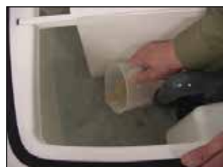
Spreading the separating agent
